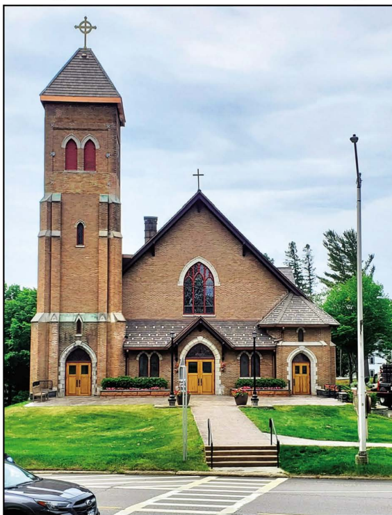
(Left) Parishioners say St. Agnes Church in Lake Placid 'finally looks finished' after the installation of a 14-foot steeple topped with an 8-foot Celtic cross. (Right) The structure was constructed in the church parking lot and then hoisted into place by a 180-foot crane.
