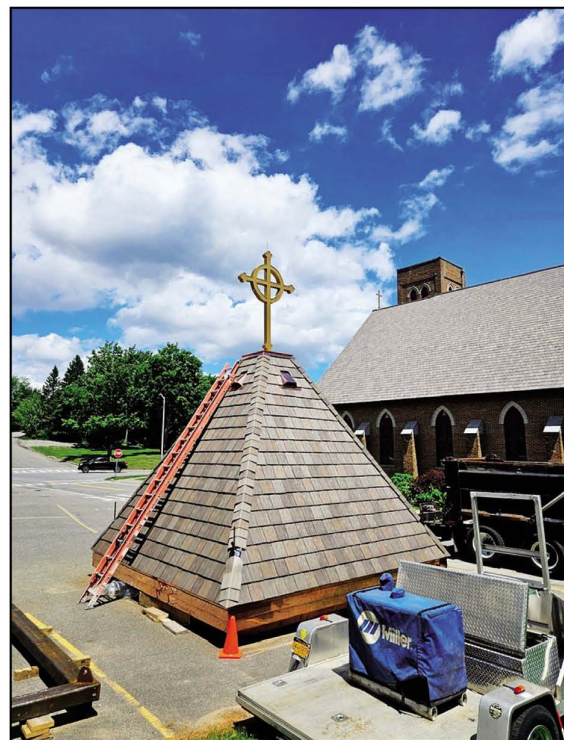
(Left) Parishioners say St. Agnes Church in Lake Placid 'finally looks finished' after the installation of a 14-foot steeple topped with an 8-foot Celtic cross. (Right) The structure was constructed in the church parking lot and then hoisted into place by a 180-foot crane.
